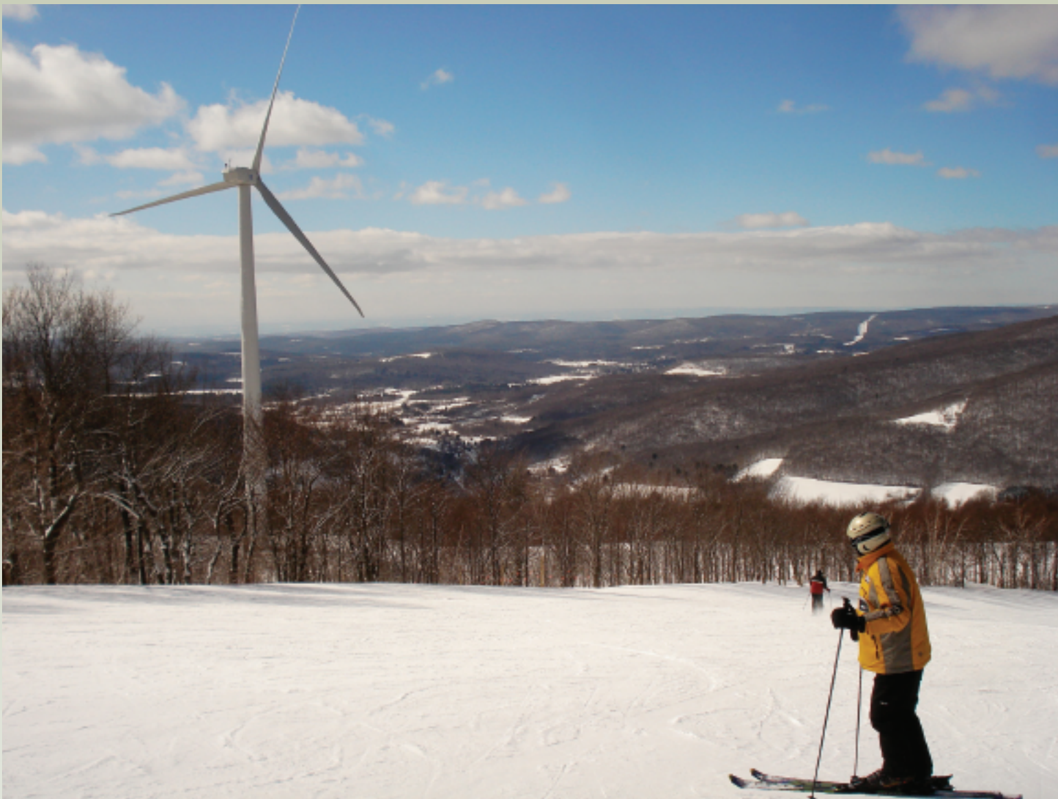
Jiminy Peak's wind turbine generates cost savings for the resort while benefitting the environment.
